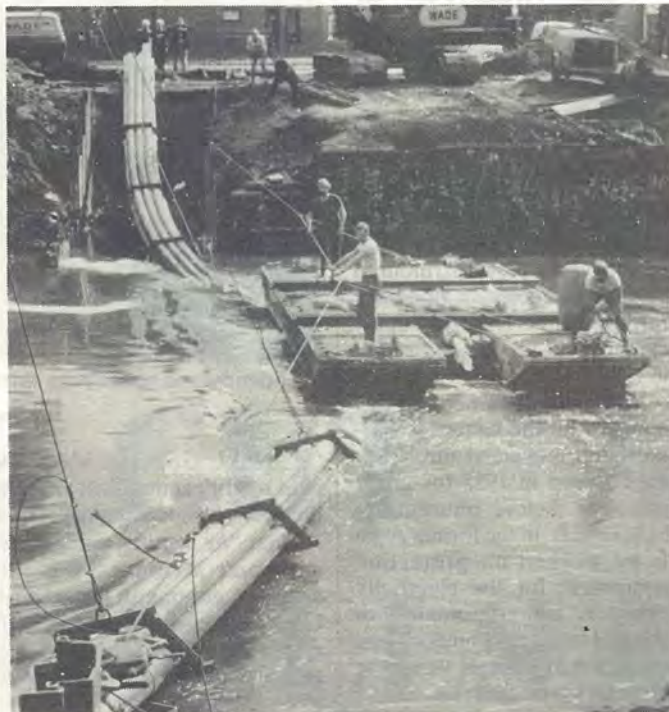
The burst of activity over, and the pipes are correctly sunk into position, with the ends out on to either bank. In the background, the coal conveyor bridge which houses the present cables.
