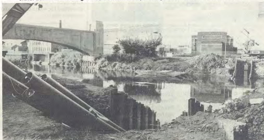
The burst of activity over, and the pipes are correctly sunk into position, with the ends out on to either bank. In the background, the coal conveyor bridge which houses the present cables.
